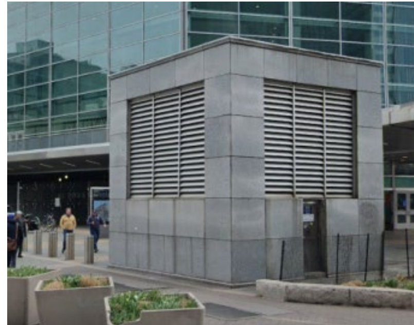
One of four ventilation structures for the Battery Park Underpass
