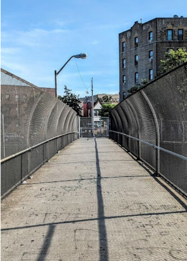
Existing Condition of Olmstead Ave Footbridge
