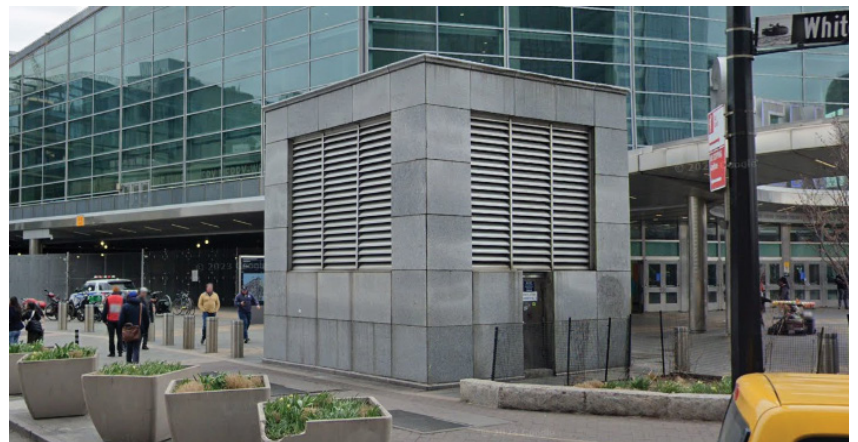
Ventilation structure for the Battery Park Underpass (Google Street View, March 2023)
